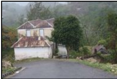
Plate 446: Property House/Old Police Station
