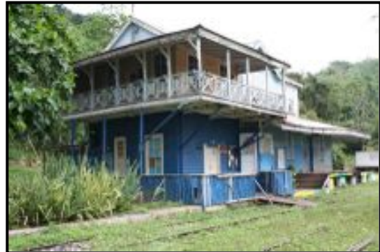
Plates 53 - 54 Railway Station
