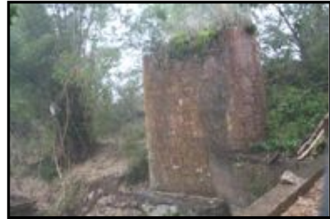
Plate 445: Old Bridge Column
