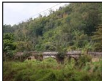
Plate 359: Bridge marks the boundary between Manchester and Trelawny
