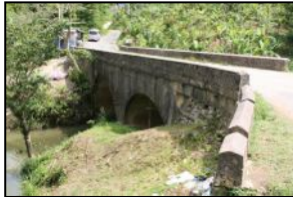
Plate 81: Marchmont Bridge over the Great River
