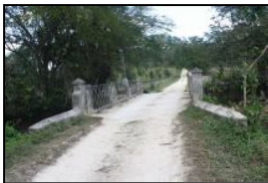
Plate 197: Bridge, Pantrepant Estate
