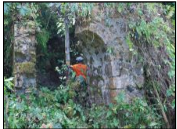
Plates 41 – 42: Structures in the works area
